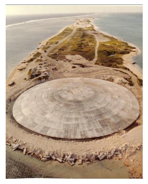
The Runit Dome was constructed in 1979 to cover 111,000 cubic yards of radioactive debris created from 12 years of nuclear tests in the Marshall Islands. (Wikimedia Commons/US Defense Special Weapons Agency)
