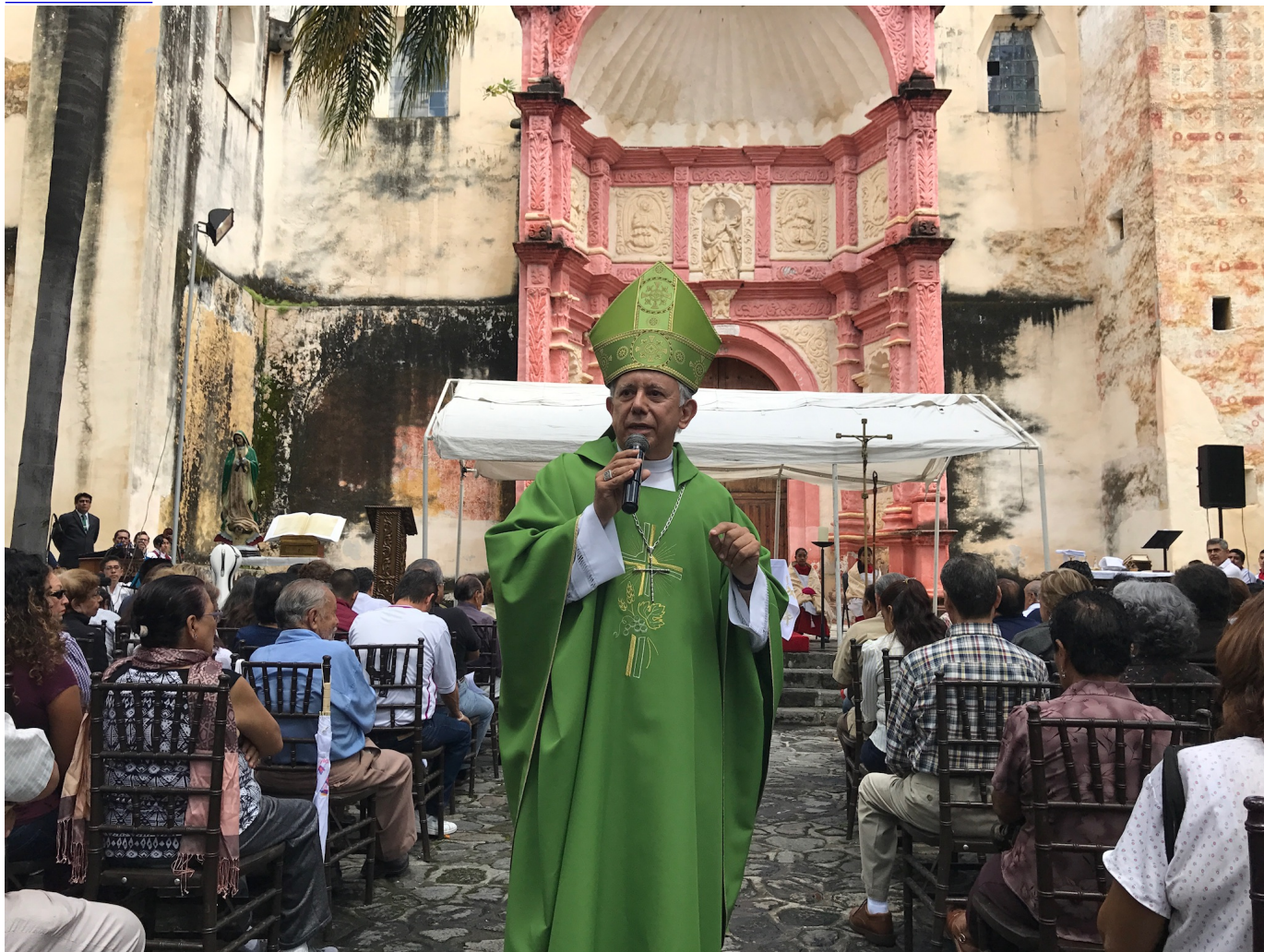
Bishop Ramon Castro Castro of Cuernavaca, Mexico, celebrates Mass Sept. 24 outside the city's cathedral, which dates to the 1500s and was badly damaged by the Sept. 19 earthquake in Mexico. (CNS/David Agren)
