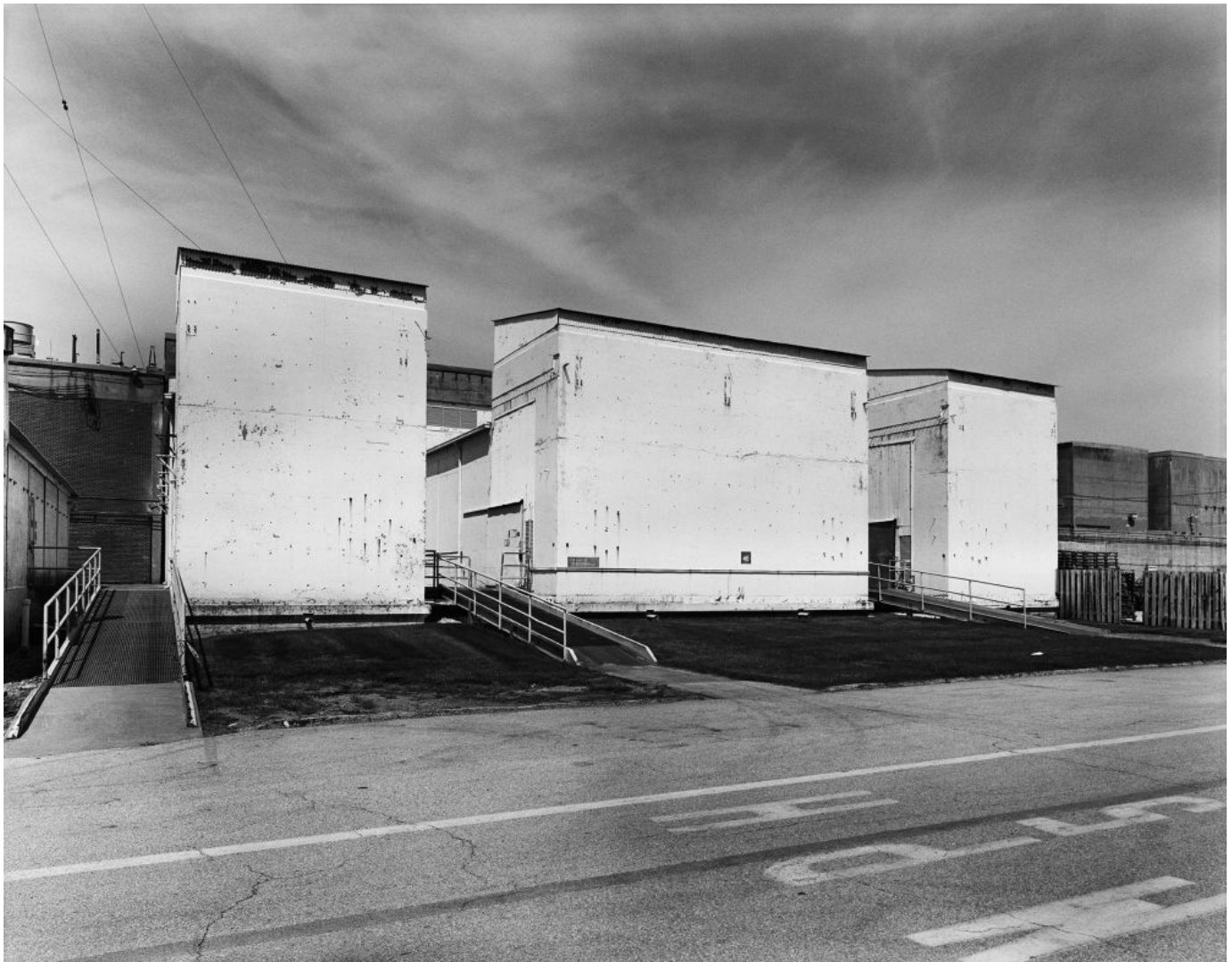
Test cells at the Kansas City Plant, 2013 (Historic American Engineering Record, U.S. Department of the Interior/Richard Welnowski)
