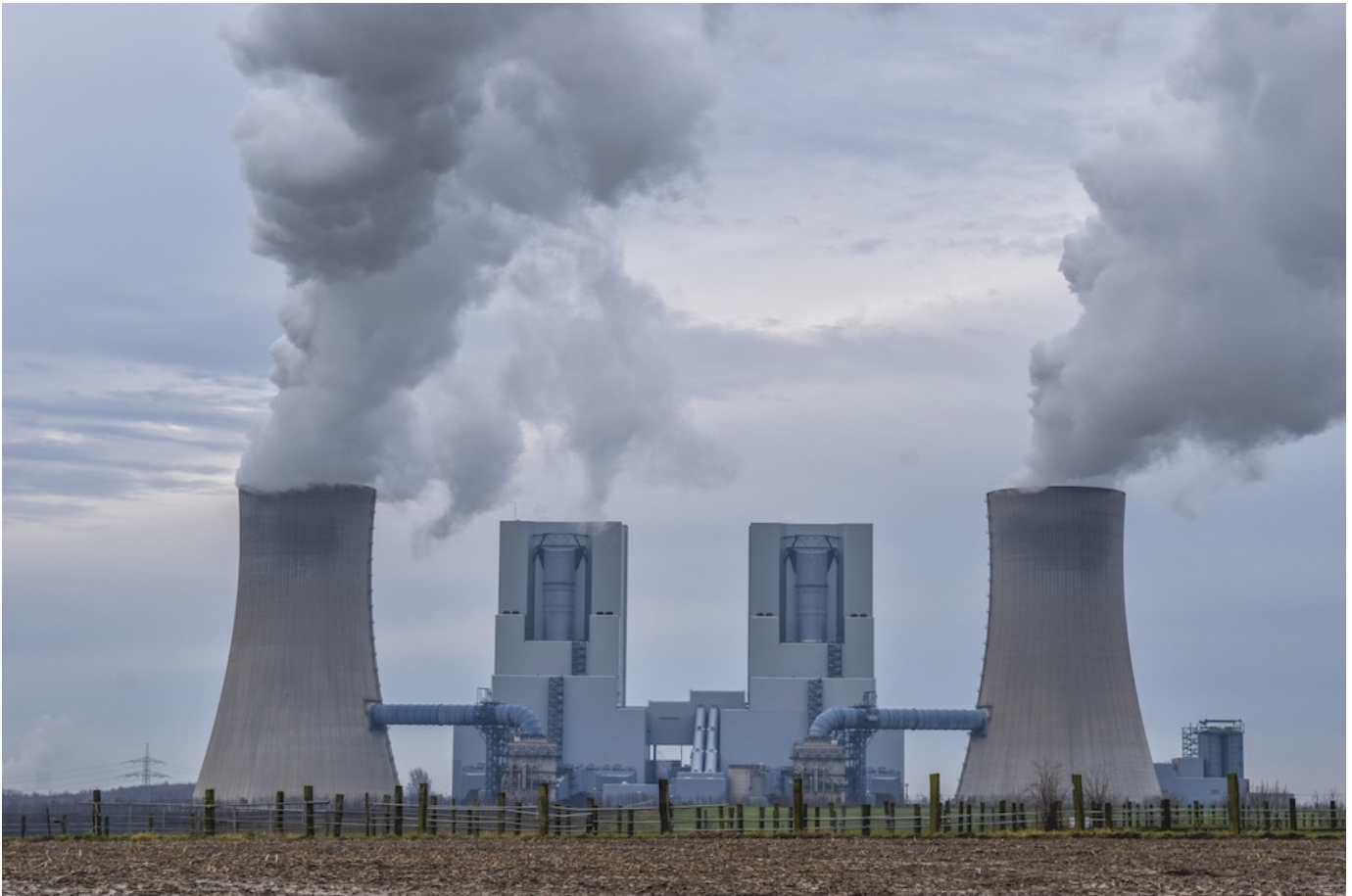
Coal-fueled power plant (Pixabay/Michael Gaida)
