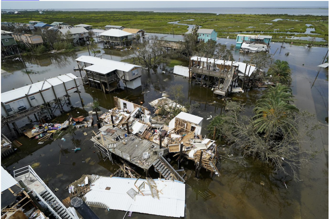
The remains of destroyed homes and businesses are seen in the aftermath of Hurricane Ida in Grand Isle, Louisiana, Aug. 31. (AP/Gerald Herbert)
