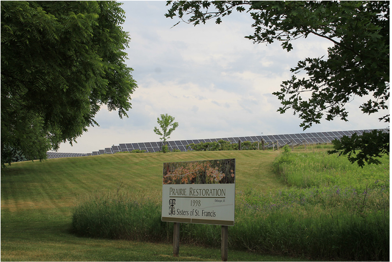
An array of 2,600 solar panels in the background of a restored prairie area at the motherhouse of the Sisters of St. Francis, in Dubuque, Iowa. (EarthBeat photo/Brian Roewe)
