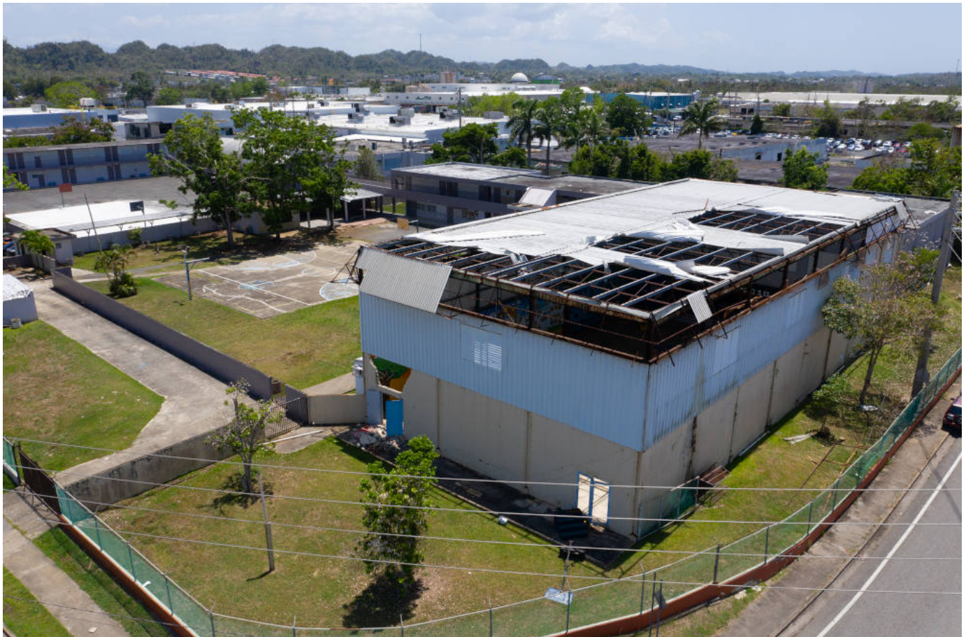
The damaged gymnasium of Colegio Nuestra Señora del Rosario in Vega Baja, Puerto Rico, in 2019. The school was damaged in 2017 by Hurricane Maria. (RNS Photo/courtesy of Catholic Extension.)
