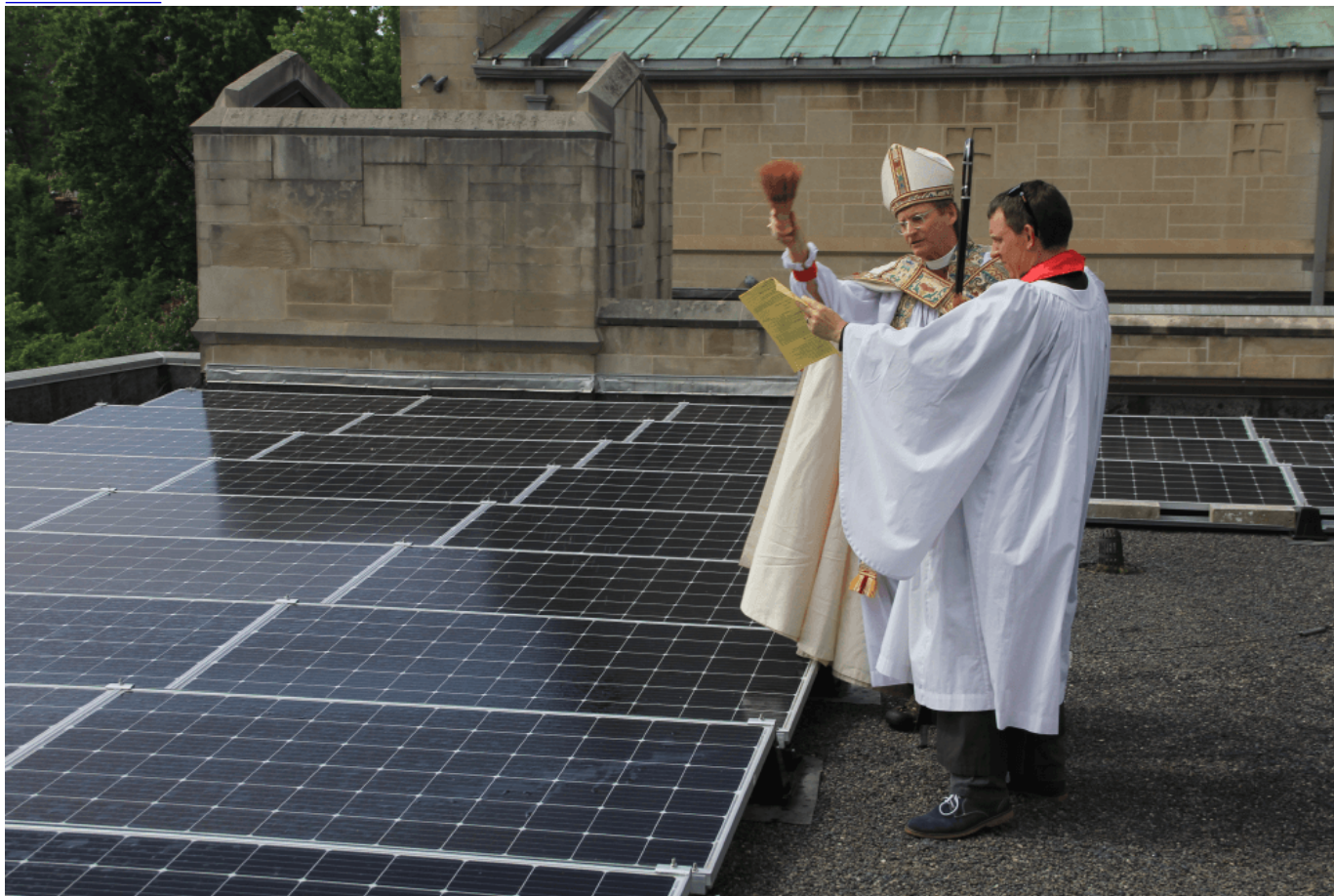
Former Pittsburgh Bishop Dorsey W.M. McConnell and Rev. Noah H. Evans bless the solar panels installed at St. Paul's Episcopal Church in Mt. Lebanon, Pennsylvania. (Courtesy St. Paul's Episcopal)
