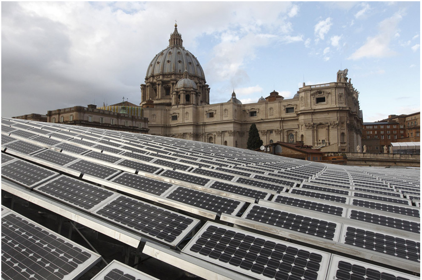
Solar panels are seen on the roof of the Paul VI audience hall at the Vatican in 2010. (CNS/Paul Haring)
