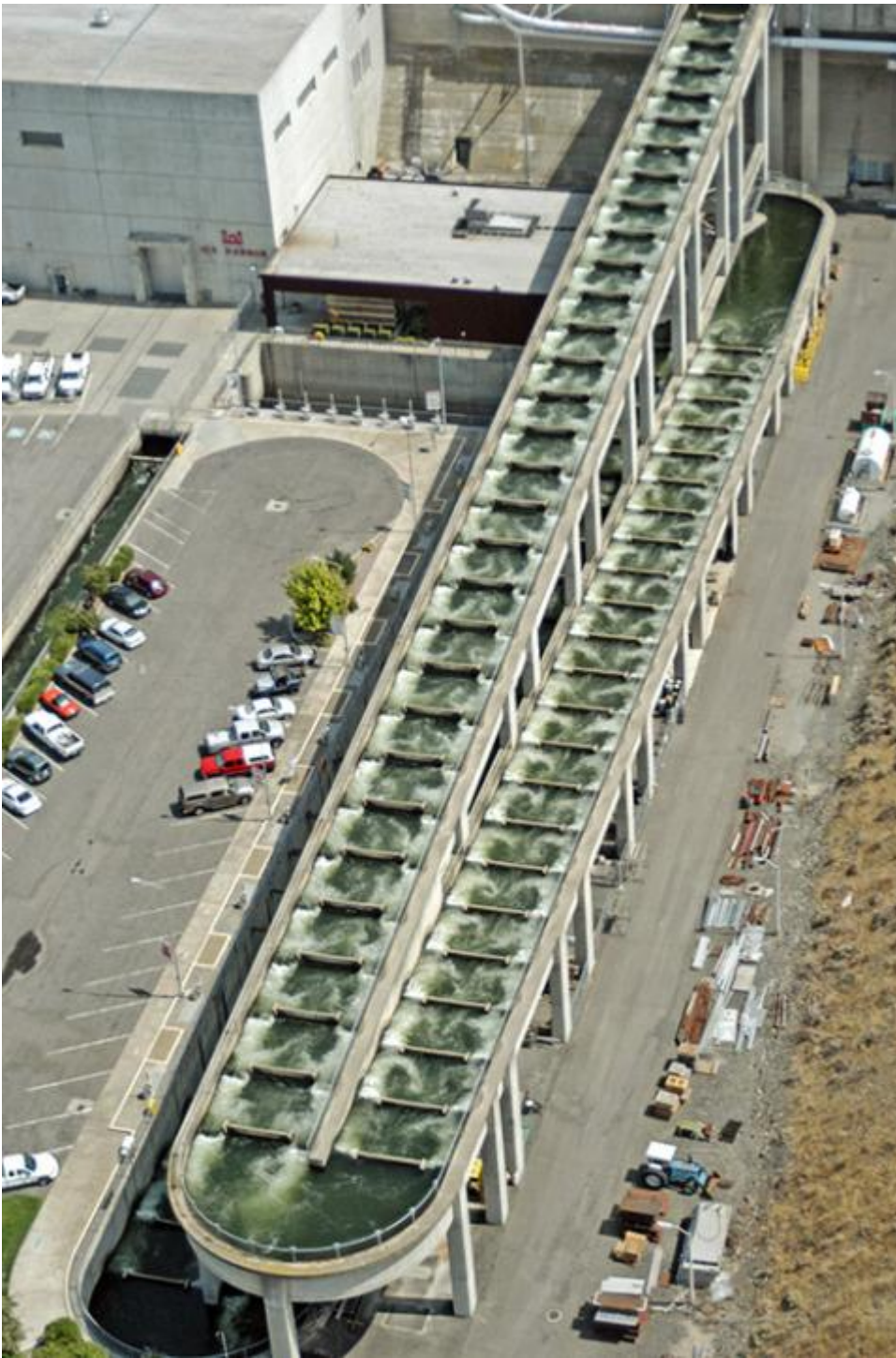
A fish ladder at Ice Harbor Dam on the lower Snake River in Washington (Wikimedia Commons/Bonneville Power)
