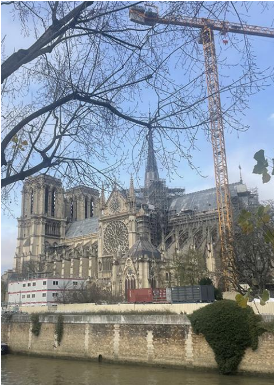
Notre Dame Cathedral as seen on Dec. 1 in Paris, still under construction ahead of its Dec. 8 inauguration Mass (NCR photo/Christopher White)
