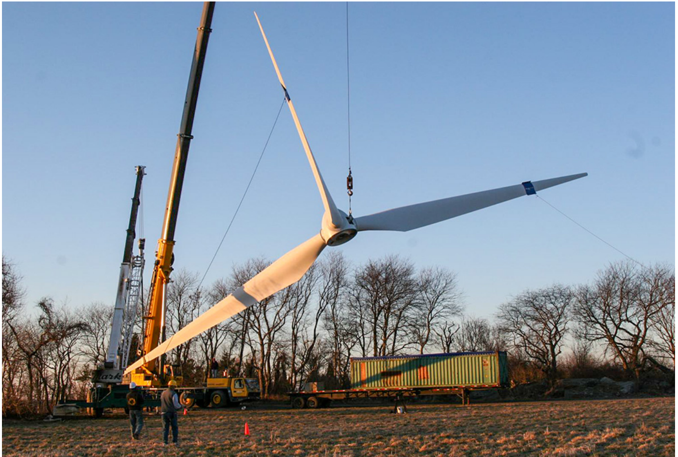
The blades of Portsmouth Abbey's wind turbine during the erection of the wind turbine in March 2006 (Courtesy of Joseph Byron)
